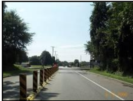
Example of Median Barriers
