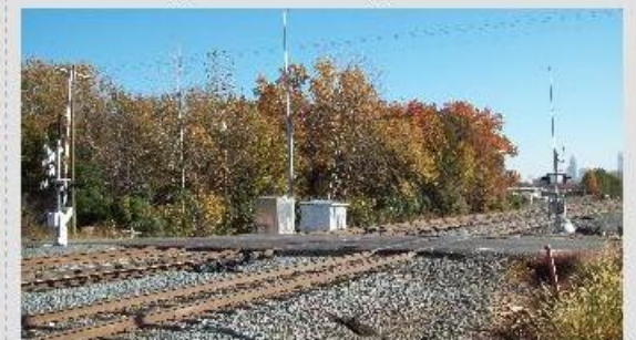
Looking East along NS Tracks
