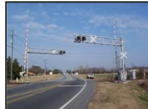
Example of gates, signs and flashing lights
