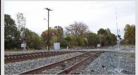
Looking West along NS Tracks
